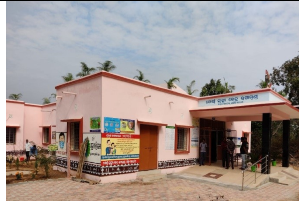
Construction of IPD at Bhagamunda CHC, Keonjhar
