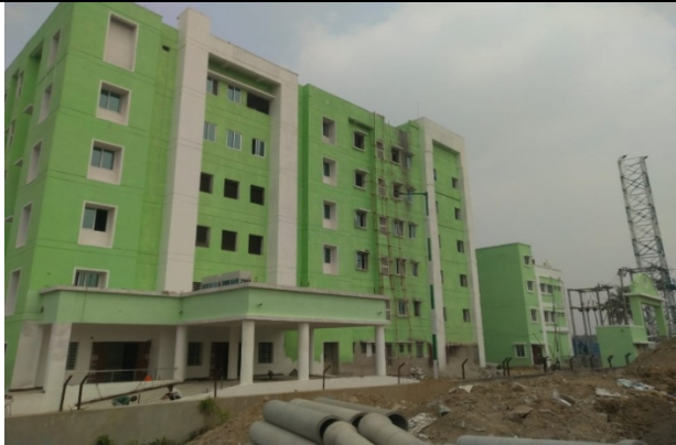
Construction of DWH & 100 Bedded MCH at DHH Kendrapara
