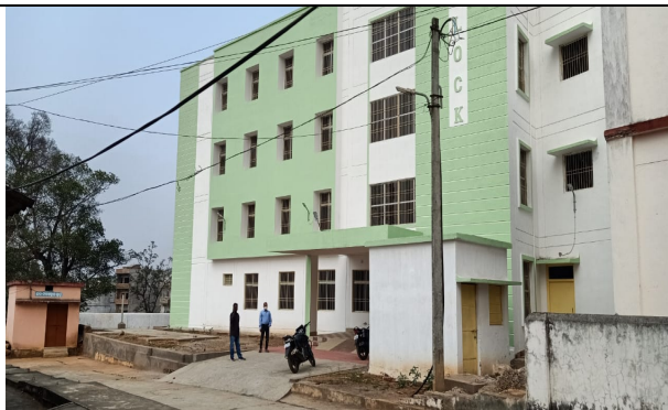
Const. of 50 Bedded IPD Building at SDH Baliguda, Kandhamal
