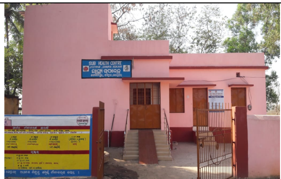
Construction of SC at Jyotipur, Keonjhar
