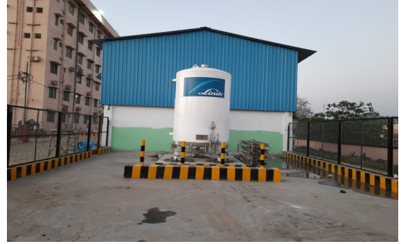
Construction of L.M.O. at Medical College & Hospital, Balasore
