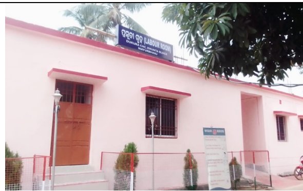
Const. of Labour Room at CHC Dukura, Mayurbhanj
