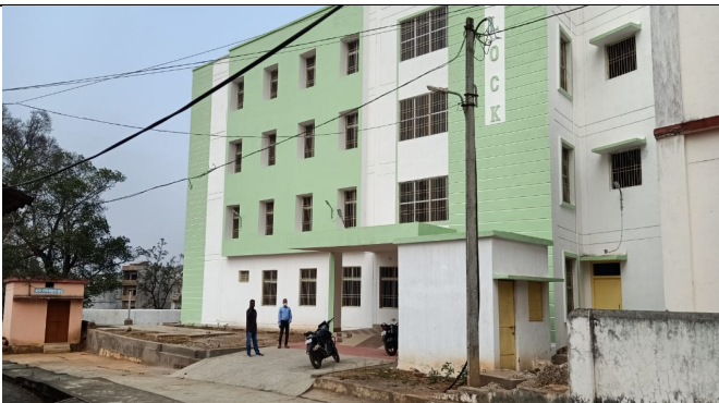
Const. of 50 Bedded IPD Building at SDH Baliguda, Kandhamal
