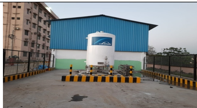
Construction of L.M.O. at Medical College & Hospital, Balasore
