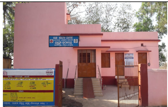
Construction of SC at Jyotipur, Keonjhar
